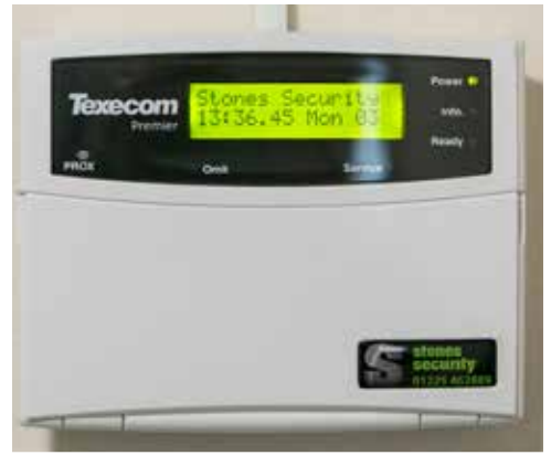
FIRE ALARM - Install
