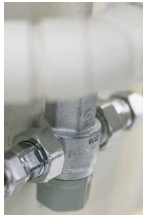
HEAT REGULATED VALVE - Pupil Safety
