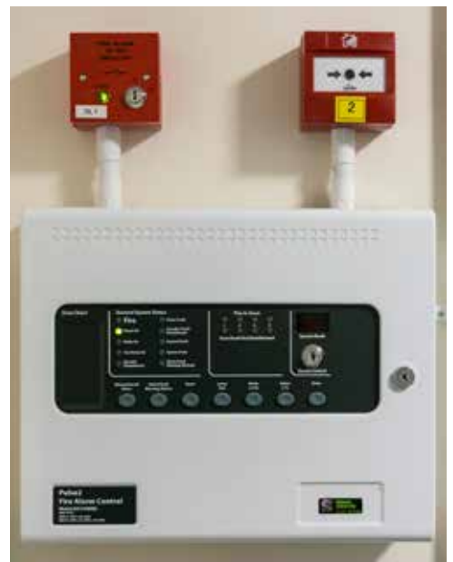
FIRE ALARM Install
