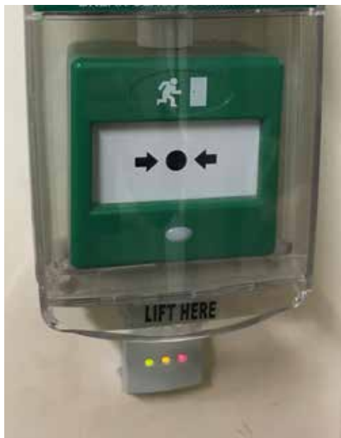
ACCESS CONTROL Main Entrance Door
