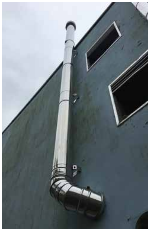
EXTERNAL BOILER FLUE - Installation
