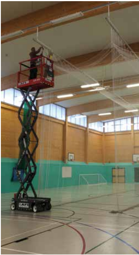
GYMNASIUM High Level Repairs
