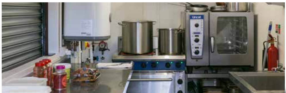
COMMERCIAL KITCHEN - Design & Build
