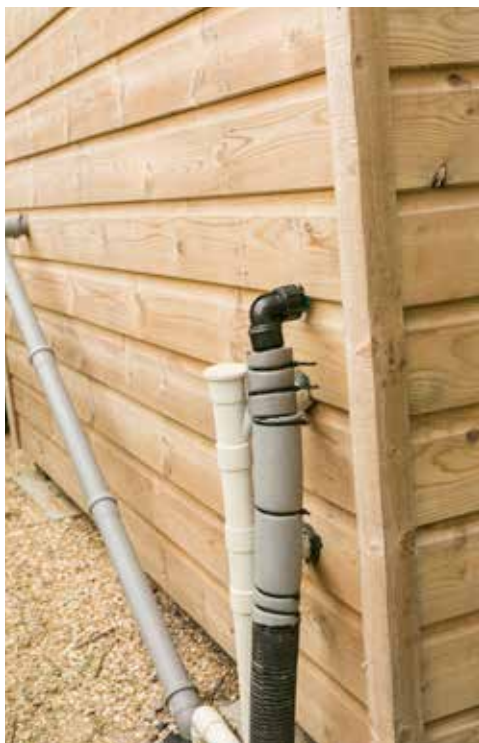
COMMERCIAL KITCHEN - Services
